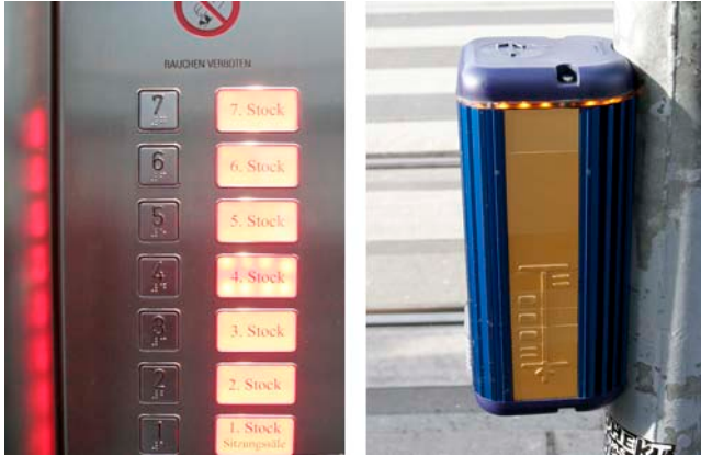
Figure 1. Braille labels inside an elevator (left) and an audible device at a pedestrian crossing that promotes its location and provides further information through tactile coding (right).
